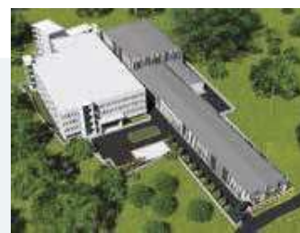
Outlook of our Factory Premises Under Renovation
